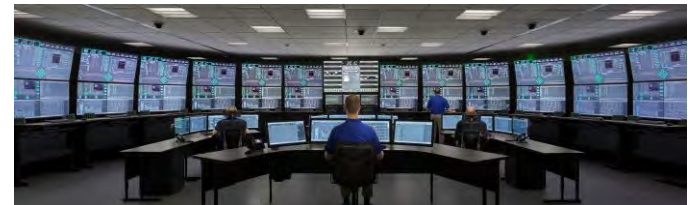
NuScale Control Room Simulator
