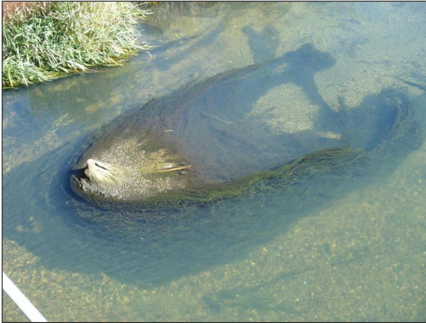
Photo 3. Algal growth on a vertical pipe, part of stream gaging equipment at Becker Line Road, Sept. 14, 2016.
